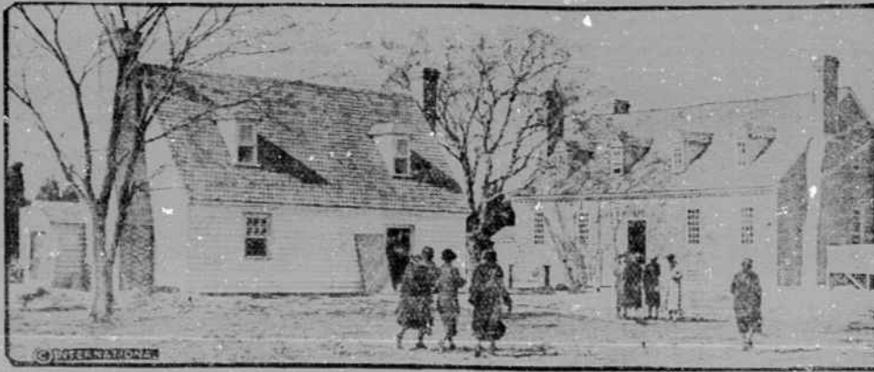
Kitchen and main house of the restored birthplace of George Washington, which is rising from the fire ruins of 150 years ago. The beautiful estate in Westmoreland county, Virginia, is being reconstructed by the government to form an almost perfect reproduction of the house and grounds as they were during the youth of the first President. The work will be completed in time for the George Washington bicentennial in 1932.
