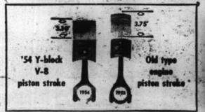
LONGER ENGINE LIFE. Both new Ford engines are of short-stroke design. This means pistons travel less distance. Naturally, there is less friction and less wear. In both engines overhead valves have a free-turning feature which allows them to rotate to cut down wear.
