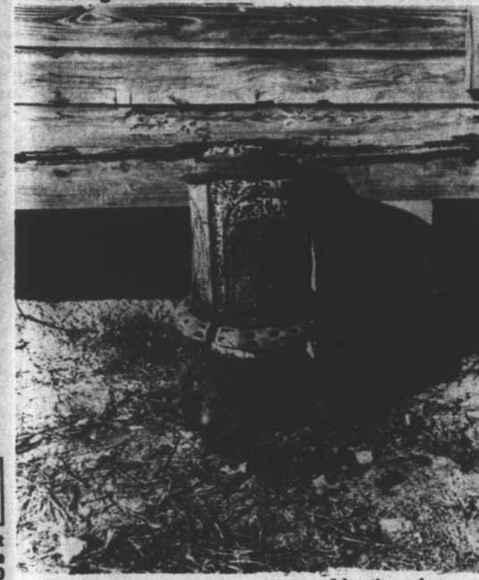
This heater was completely unusable. Recipient had no means of heating whatsoever before receiving new heater.
