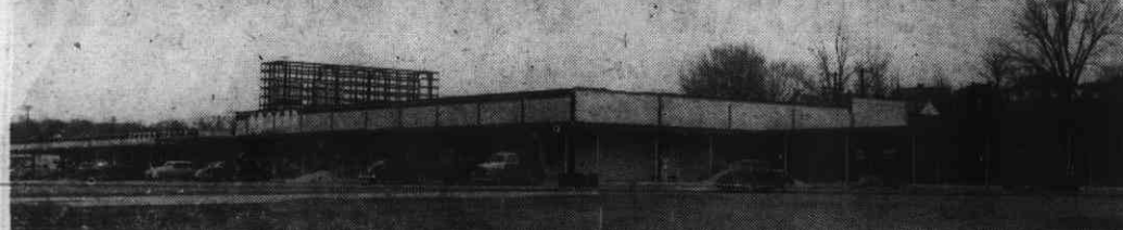
Pictured above is the new Kroger Store which will be opened in Durham on April 5. Located in the newly constructed Forest Hills shopping center, the mammoth store will contain floor space of 18,000 square feet, making it one of the largest super markets in the State. Among its other features will be air conditioning and modern furnishings throughout.
