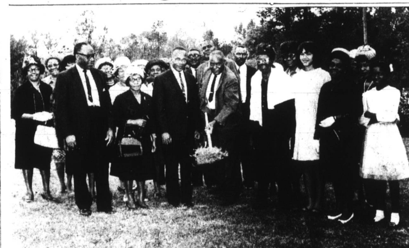
GROUNDBREAKING for the erection of a new edifice for the Ebenezer Baptist Church was held on the site in the 2200 block of Alston Avenue Road here, Saturday, May 29. Participating in the memorable occasion were the pastor, Rev. J. A. Brown, several officers and members of the church. Rev. Brown is shown at the left in the front of the picture. The first shovel of dirt was dug by Howard Williams, Chairman of the Deacon Board, as shown in the center of the above photo. (Photo by Purefoy)
