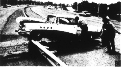
A steel median barrier on the Thornton Freeway in Dallas kept driverless car from entering other side of the road.
