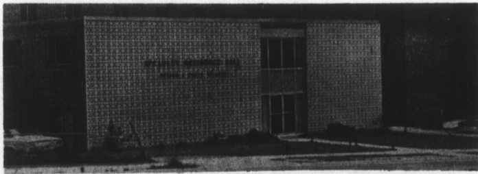
McCauley Residence Hall for Women. Each Room Individually Heated and Air Conditioned.
