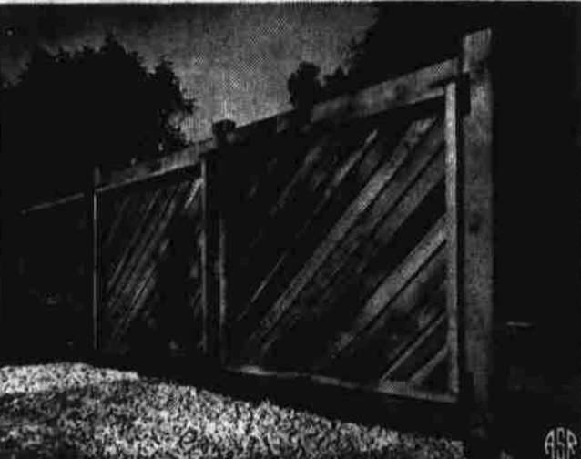
BEAUTIFUL AND DURABLE —Diagonal 1x4 redwood boards in picture-frame panels make for an interesting, functional barrier between patio and service areas. Sturdy Construction Common, knot grade redwood was used by the fence designer, a landscape architect, for its beauty and durability.
