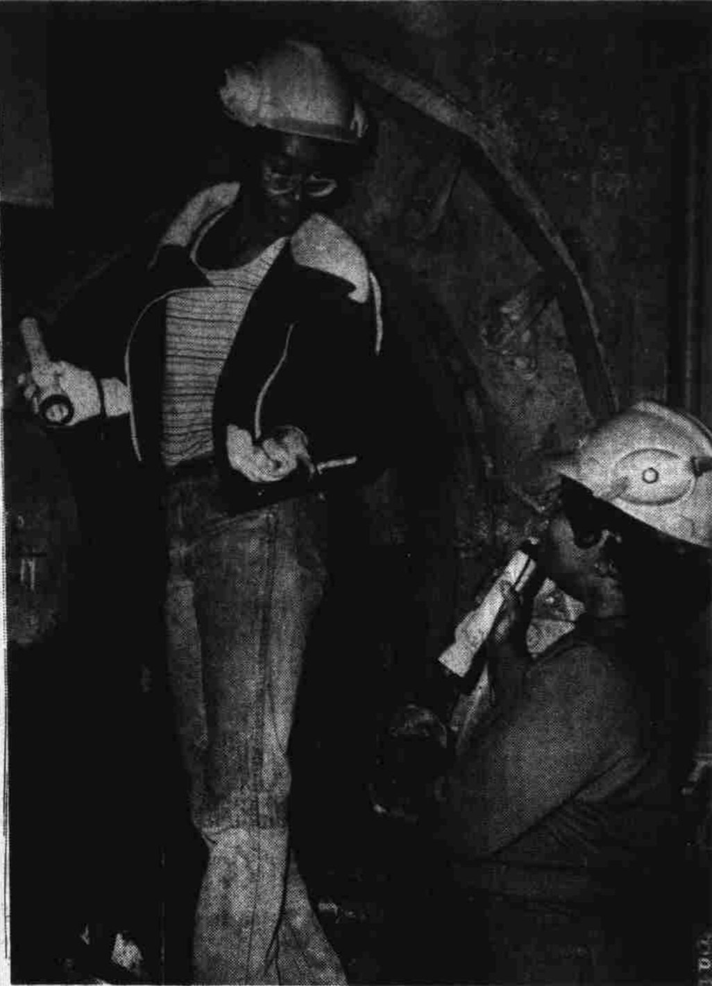
WOMEN IN HARD HATS —Linda Brown, left, consults with Ada Parker about the lubricating oil and the cooling mechanism on the giant fans which blow air into the boilers at Con Edison's Hudson Avenue electric generating station in Brooklyn. Mechanics for the utility, they have jobs once considered "for men only."
