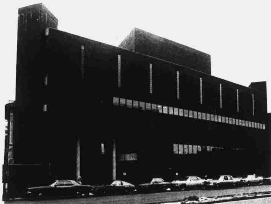
The New Home of The Schomburg Center for Research in Black Culture (515 Lenox Avenue, New York City); The five story red-brick building designed by Bond, Ryder & Associates, occupies the entire block between 135th and 136th Street along Lenox Avenue. Afro-American architectural history was the guide in the design of the central rooms and the second-floor Rare Books, Manuscripts & Archives section has walls paneled in sapele wood from Nigeria.
