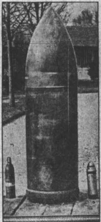
This tremendous shell is one of those fired by the giant 42-centimeter howitzer of the German army. It fell in soft dirt near Verdun without exploding and was dug up by the British. Beside it, on the left, is a French 15-mm field gun shell, and on the right a German 77-mm shell, each of which is about three inches in diameter. The big shell is five feet long and weighs almost a ton.
