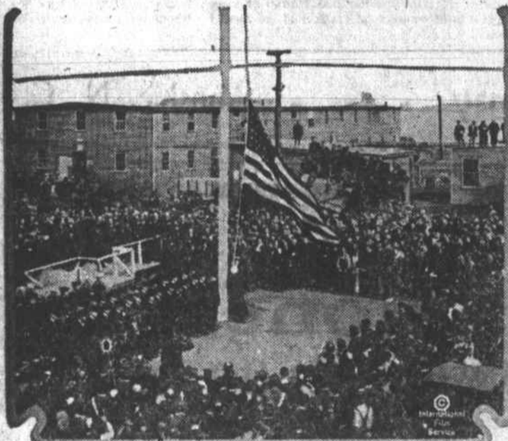
The Fore River shipyard having received large orders from the United States government for the construction of warships, merchant ships, and scores of torpedo boat destroyers, it has been found necessary to enlarge the plant and they have therefore taken the old government aviation field at Squantum and are turning it into a huge shipbuilding yard at the cost of $28,000,000. Photograph shows the Stars and Stripes being raised at the new yard. Naval men and thousands of employees took part in the ceremonies.
