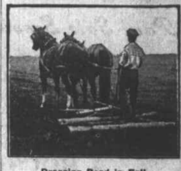
Dragging Road in Fall.
