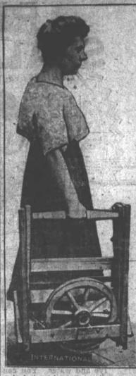
At last we have the rolding wheetparrow. When not in use it can be folded up and stored away in a closet. The folding wheelbarrow is the invention of a French mechanic. The photograph shows the wheelbarrow folded and ready to be stored for the
