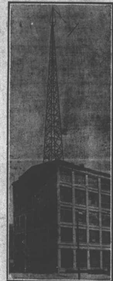
One of the Antenna Towers of WGYY, Radio Broadcasting Station of General Electric Company.
