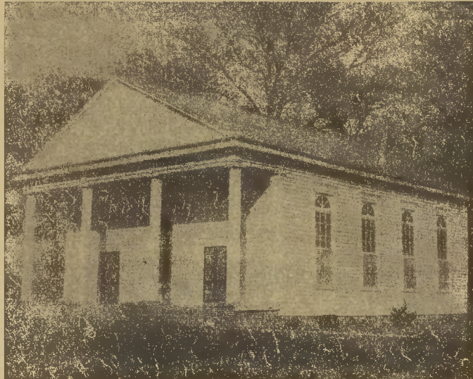
PLEASANT GROVE—One of Hertford's oldest church buildings is the plain frame meeting-house of Pleasant Grove Baptist Church. Interesting architecturally for its severe, classic lines, the building is striking for its high windows. The building has changed little since ante bellum days when it was built. The building has been the scene of several associational meetings of Baptists, and for many years was home church for Dr. Godwin Cotton Moore, ante bellum Baptist leader who served 37 years as moderator of the Chowan Association.
