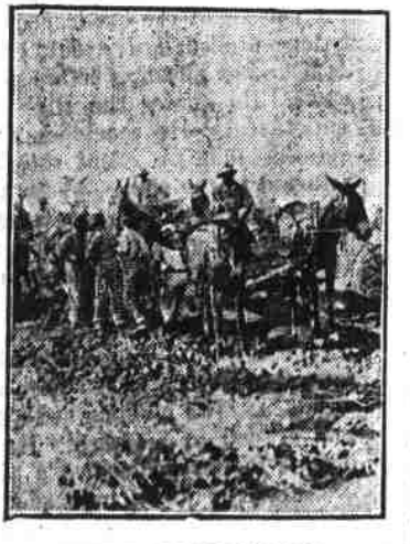
MAKING A SAND-CLAY ROAD.
