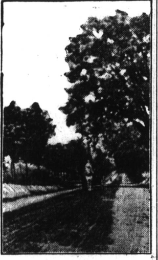
Road of Bituminous Macadam.
