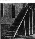
By Constructing the Outside Stairway of Concrete, a Dependable Fire Es cape Was Provided at a Nomina
