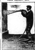
end. England, with the aid of a cemer gun. A frame of timber is bolted to-gether with expanded metal, onto gether with expanded metal, onto which is pumped by a 60 horse power motor a substantial thickness of sand and cement. This is the first building constructed in this manner in Eu
