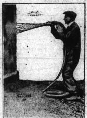
Houses are being erected in South and, England, with the aid of a cemen gun. A frame of timber is bolted to gether with expanded metal, onto which is pumped by a 60 horse power motor a substantial thickness of sand and cement. This is the first building constructed in this manner in Eu
