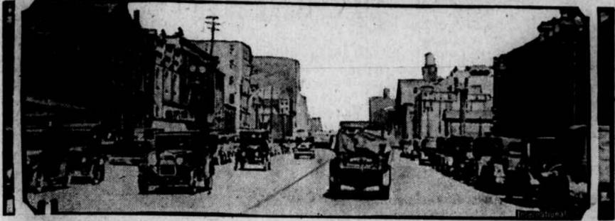
This concrete boulevard through Syracuse, N. Y., and vicinity, has replaced the famous Erie canal, now abandoned. The waterway was filled in with rubbish and dirt hauled from nearby hills and the concrete was laid on the surface.
