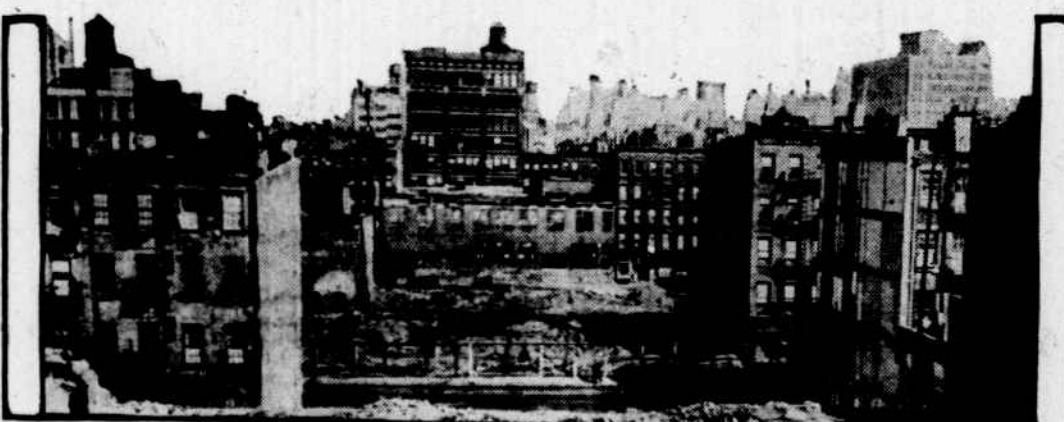
Demolition of ninety-one old houses in the Hell's Kitchen district, to make way for the Manhattan approach to the Midtown tunnel has been started. The work involves the razing of structures from Thirty-fourth street to Forty-second street, between Ninth and Tenth avenues.
