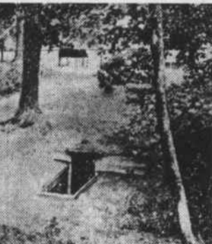
The Crater of the Mine Exploded on July 30, 1864, Showing the Entrance to the Federal Tunnel.
