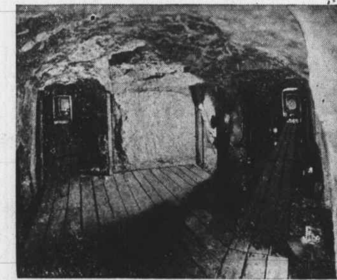
Part of the Confederate tunnel system as it is today. Apparently forgotten since shortly after the Civil war, this tunnel constructed during the long siege of Petersburg, was discovered by accident about ten years ago by a farmer clearing land. In the photograph are shown the entrances to two branches of the passage. The one on the right is nearly a mile long. The left one is 1,700 feet long. Both are about 5 feet wide and 12 feet under the surface of the ground at the entrance.
