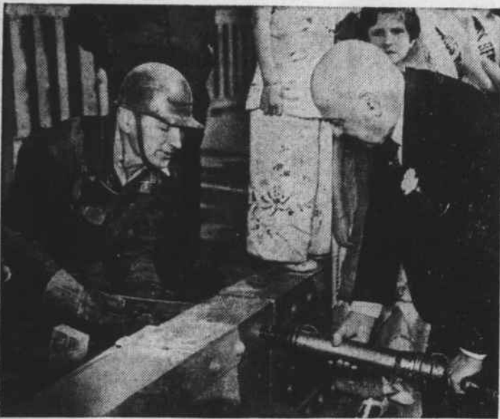
The last rivet was recently driven in the Golden Gate bridge at San Francisco. With many notables witnessing the ceremonies, a crew of iron-hatted riveters drove a golden rivet into the span, signaling completion of the structural steelwork. Mayor Rossi (right) of San Francisco aided by riveter Edward Stanley drives the last rivet.
