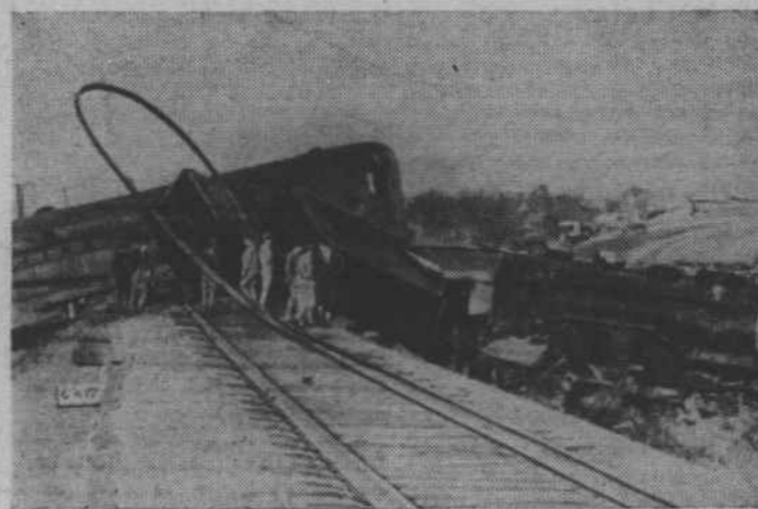
This photo shows the wrecked locomotive, tender and car of the streamlined railroad train that struck a truck near Dallas, Texas. Note the rail twisted and uprooted 30 feet in the air by the impact. Two were killed as a result of the accident.
