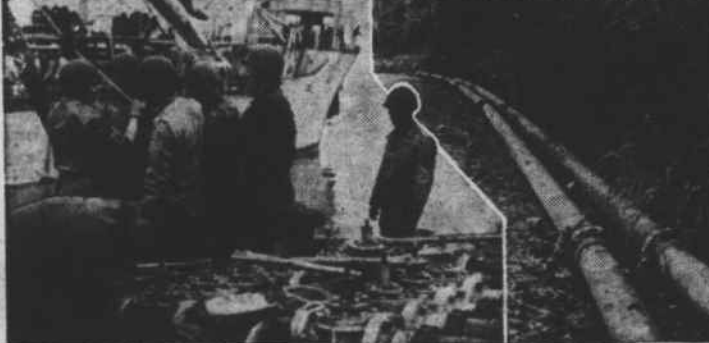
A pumping station, one of many set up along the pipeline carrying vital fuel oil in France. Upper photo shows station carefully camouflaged against air observation. Lower left, ship-to-shore line for unloading petroleum from ships. Lower right, American engineers have laid this gasoline pipeline in France, five miles inland.
