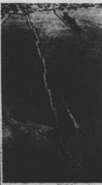
Seabee "Seven-League Boots," as shown in aerial view of the attenuated pontoon causeway, spun out by the navy's Seabees to aid in bringing additional supplies ashore during the invasion of the Philippine Islands. Seabees also built airfields.
