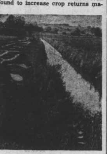
Typical New York state drainage ditch.
