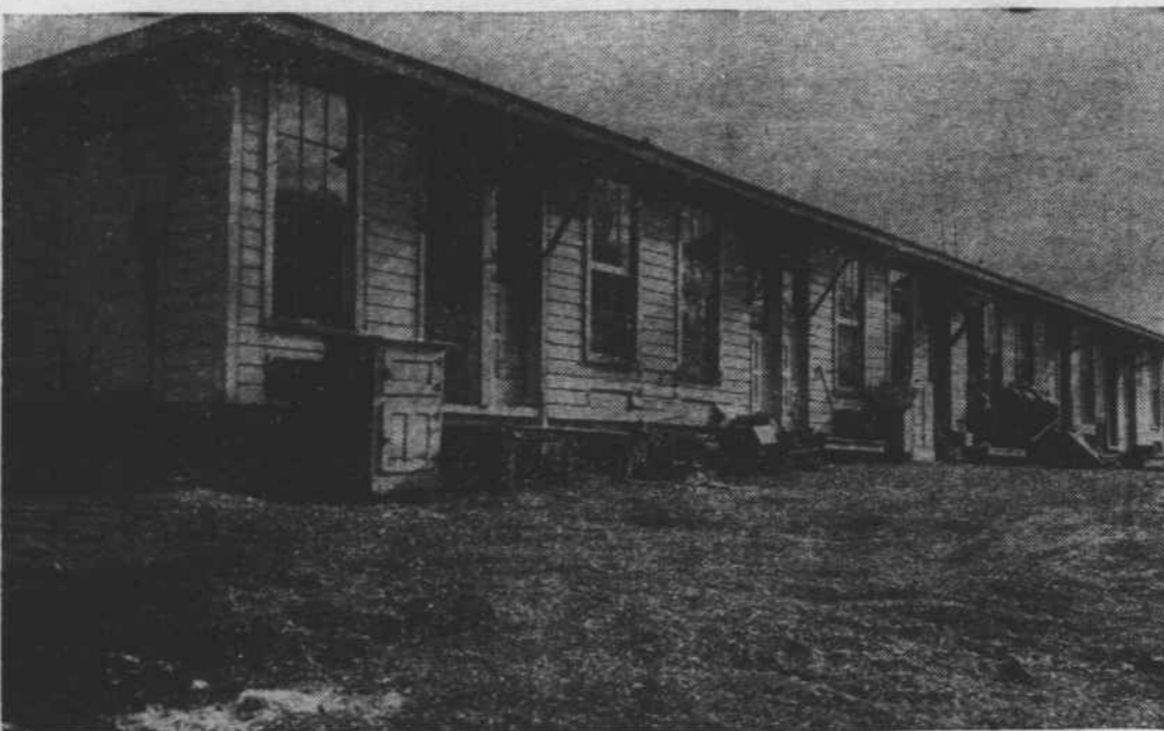
HIGH COST OF LIVING IN A CHICKEN HOUSE . . . A few weeks ago this was a chicken coop on the farm of Herbert Studebaker, Waterloo, Iowa. Today it is converted into eight one-room kitchenette apartments, with a utility room for use of all tenants. There were more takers at $52.50 a room per month than the Studebakers could handle on their poultry farm. More revenue from renting than raising chickens!
