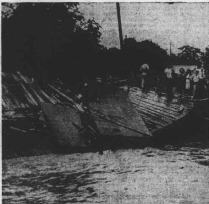
SAN ANTONIO HIT BY WORST FLOOD IN HISTORY . . . San Antonio citizens are occupied by trying to make some sort of order out of the chaos caused by the worst flood in the history of the city. Nearly a score of lives were lost and damage was reported at six million dollars. Photo shows crowd on bank looking at the wreckage of a bridge which was swept away and was washed along for a quarter of a mile by the raging flood waters.
