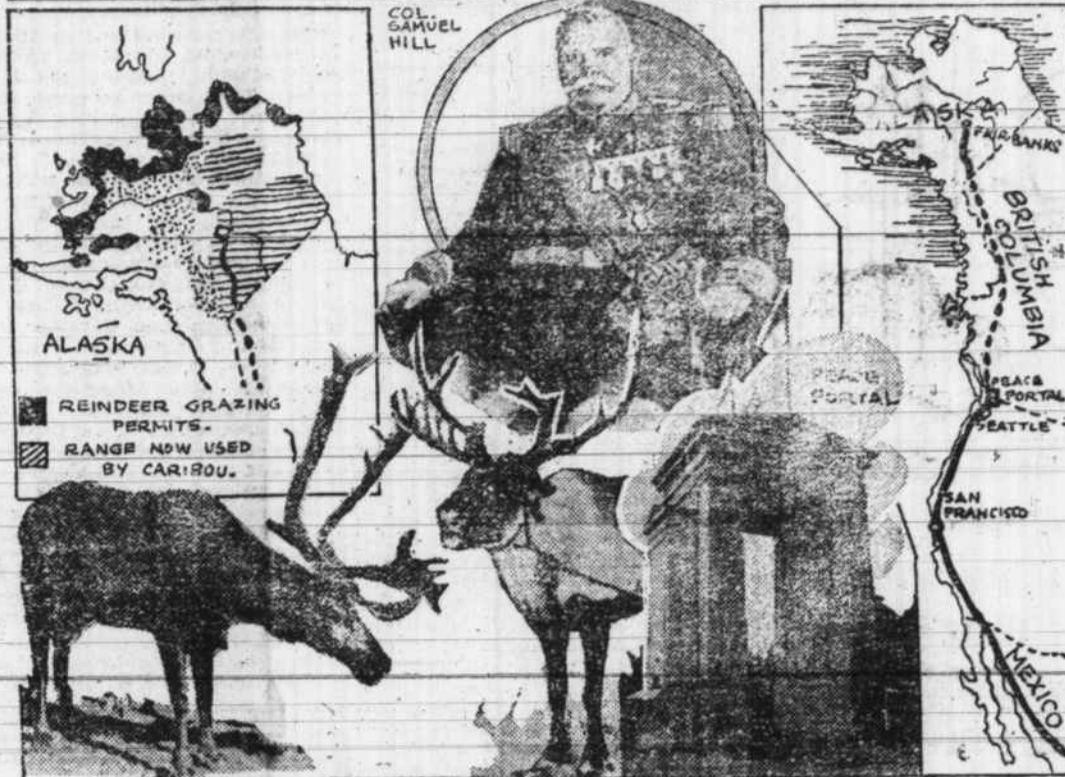
Col. Samuel Hill of Seattle, famous international capitalist and promoter of good roads, is behind the project to build the connecting link between British Columbia and Alaska which will make a continuous motor road from Mexico to the Far North. The road will pass through the Peace Portal which stands on the International boundary line. The Reindeer meat industry in Alaska is being fostered by the Government which owns great herds which serve as food for the Eskimos.
