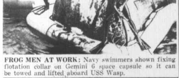
FROG MEN AT WORK: Navy swimmers shown fixing flotation collar on Gemini 6 space capsule so it can be towed and lifted aboard USS Wasp.
