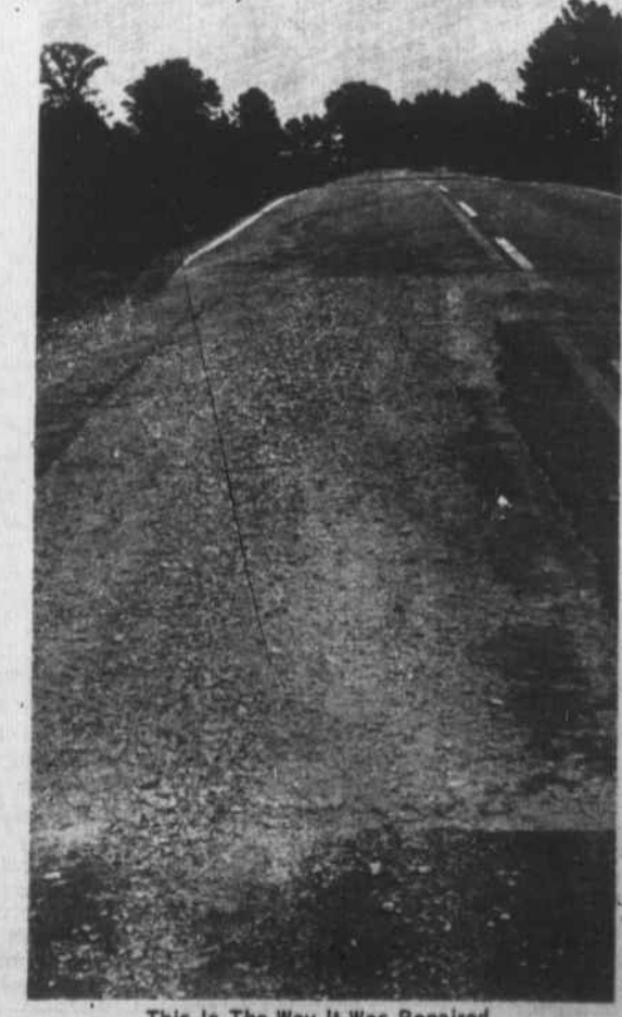
This Is The Way It Was Repaired
