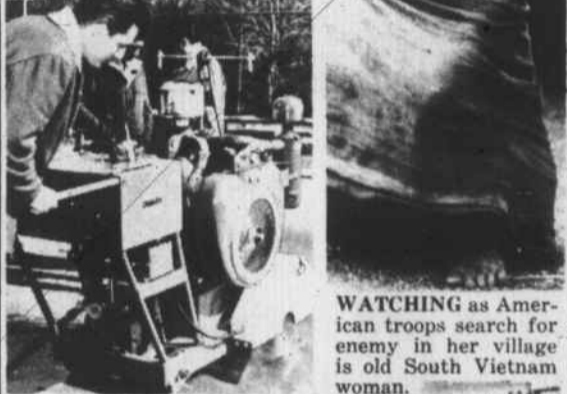
CUTTING UP: An Omark diamond-edge saw slices concrete for repair job in New York, reducing need for jackhammering.
