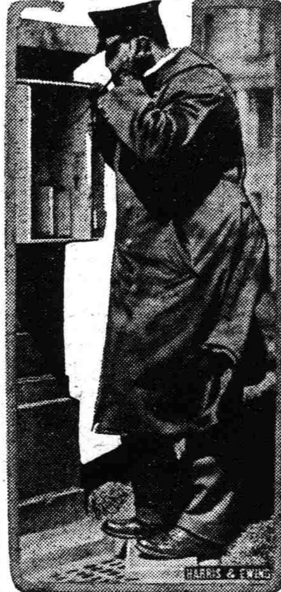
Guards at the gates of the White House have been provided with telephones connected directly with the White House switchboard. Each gate is in instant communication with all the forces which guard the president.
