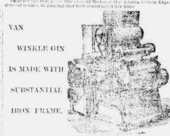
THE RIBS ARE MADE OF THE BEST CHILLED IRON AND MOST Improved PATTERN. The SAWS of BEST ENGLISH Steel AND NEEDLE POINTED. live of making a machine work for general results.
