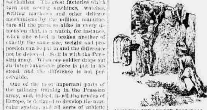
HOISTING THE TWENTY-FOOT WALL.
