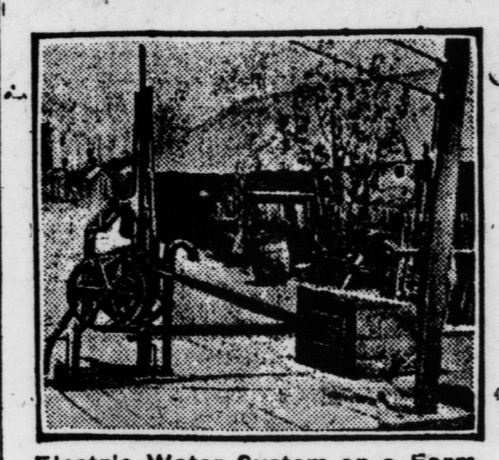
Electric Water System on a Farm. Motor is Inclosed in Box.
