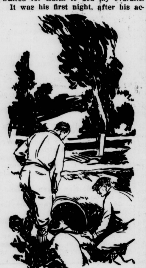
Made an Examination of the Culvert.
