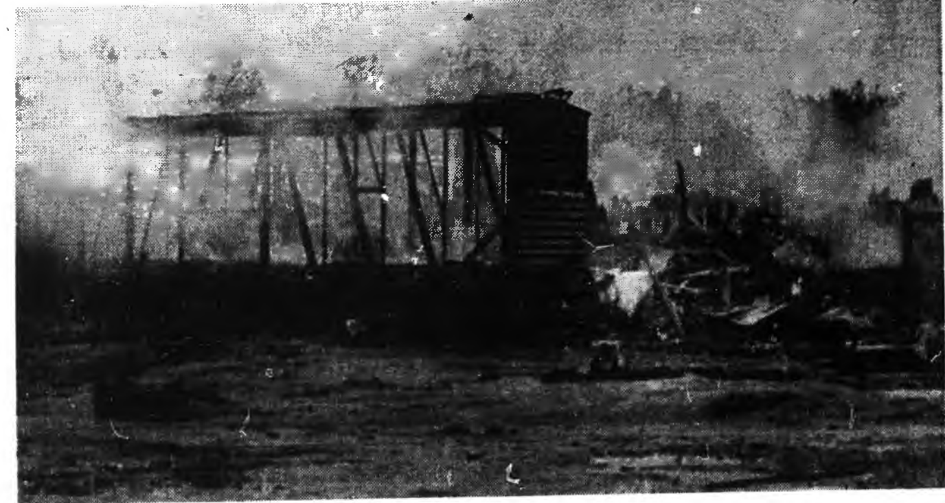
This box car which stood beside Home Chair company plant was still burning Thursday as mute evidence to the scope of the flood disaster
