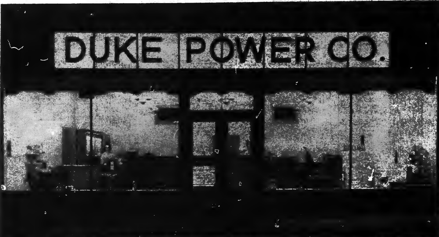
Formal opening of Duke Power company's new office at 367 Ninth street will be held on Thursday, January 16th, three to 9:30 P. M. The public is cordially invited to the formal opening for inspection of the new offices, showroom, demonstration room and other departments designed to increase efficiency to customers.
