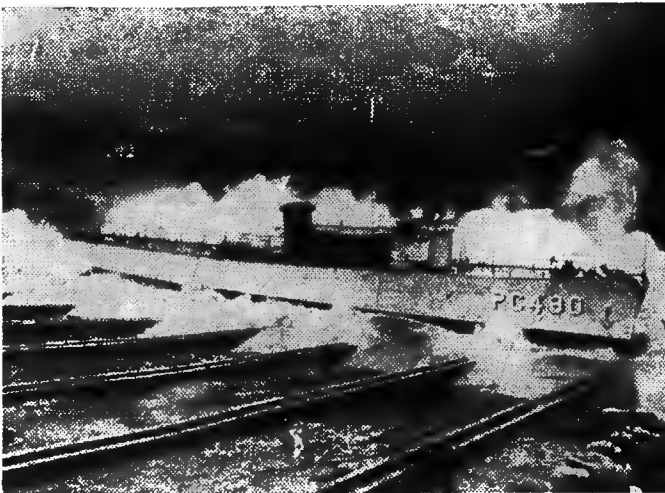
The submarine chaser, PC-490, sliding down the ways in a broadside launching at the Neville Island yards of the Drave corporation, Pittsburgh, Pa. It is the first of 15 such craft being built here for the navy, which will travel down the Ohio and Mississippi to join Uncle Sam's growing forces at sea.
