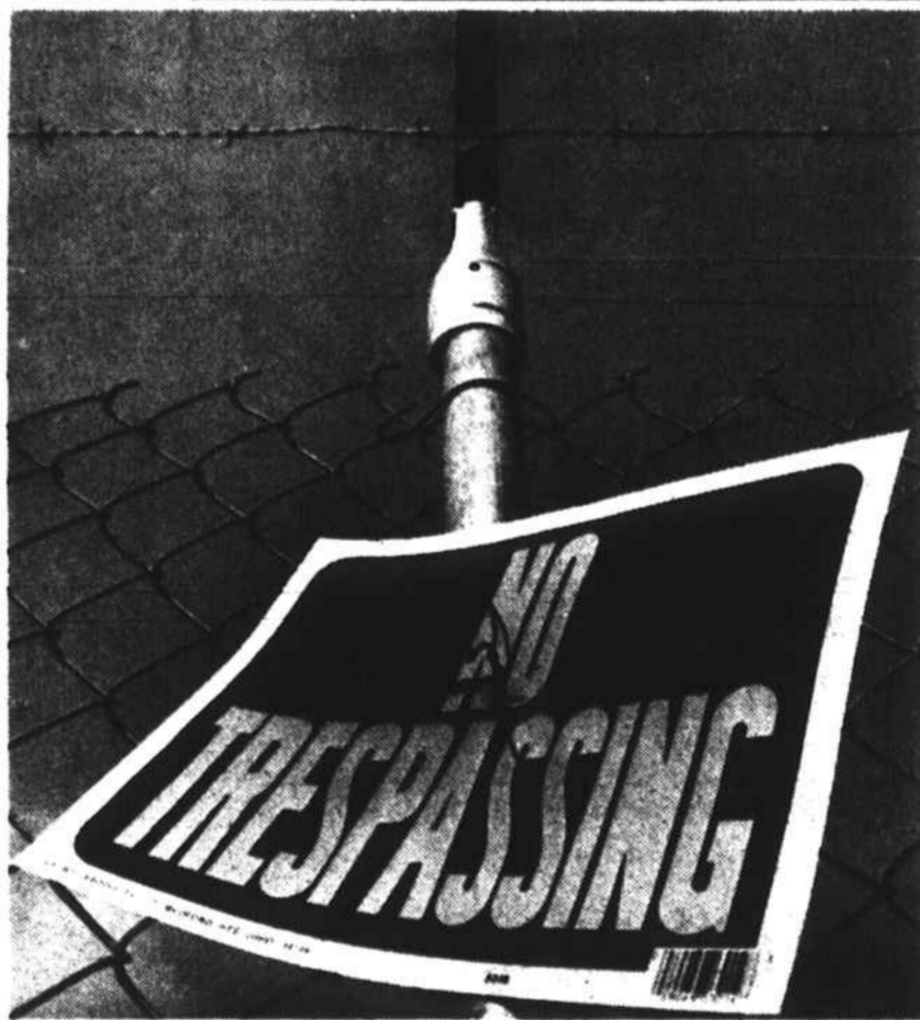
Barbed wire and no trespassing signs greet passersby at the Winston Lake Y's construction site (photo by James Parker).
