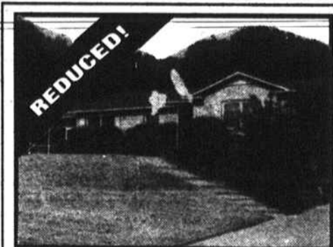
2920 SPRINGHAVEN DR.-EXCELLENT CONDITION! —3BR, 3 1/2BA, finished playroom in basement. Truly a great house w/lots of room & a beautifully landscaped yard, screened porch & deck.
