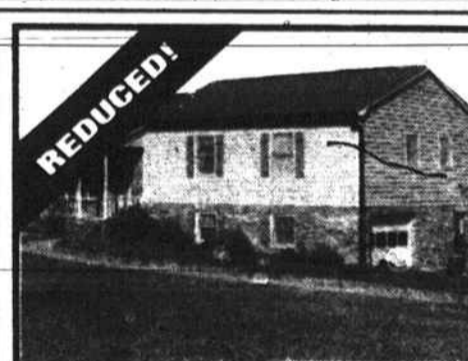
3767 DAY ROAD-WALKERTOWN DELIGHT!!! —3BR split level on a large lot. Spacious living area w/ plenty of room for a family. Bsmt gar., finished bsmt playroom, and a beautiful view off back deck.
