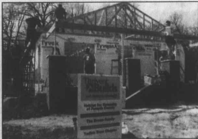
Volunteers work on the Thrivent Habitat house.
