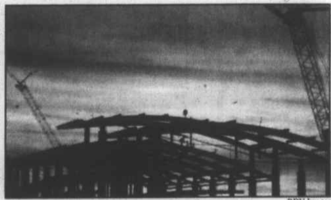
Construction is ongoing on the new terminal.
