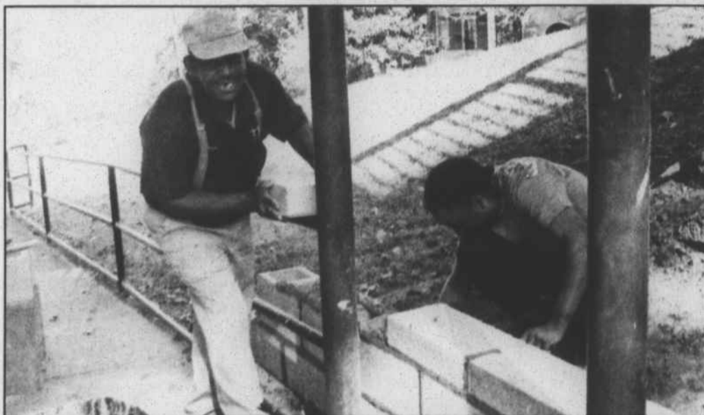
Herbert and Marcus Graham work to complete the wall.
