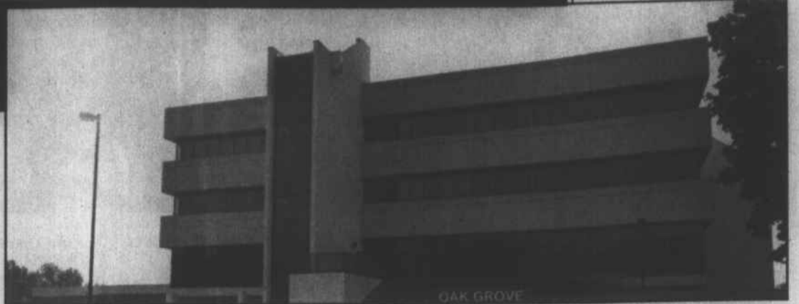
Below: A 2008 bond paid for the transformation of the school system's Career Center into Forsyth Technical Community College's Oak Grove Center. The college is depending on this year's bond to complete its renovation.
