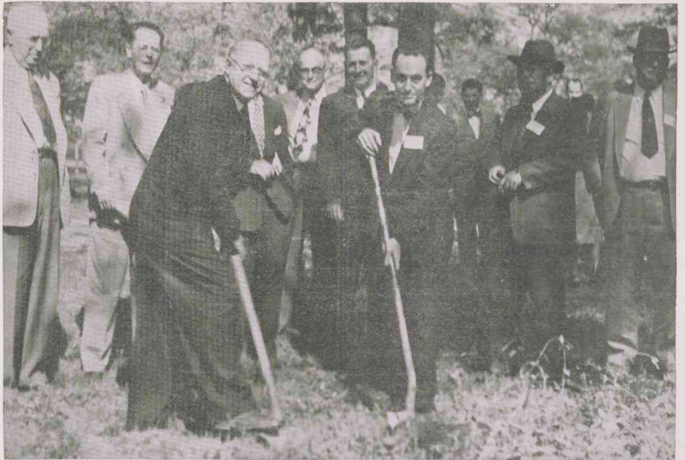
GROUND BROKEN FOR GRAPHIC ARTS BUILDING —Eastern Carolina Press Association members watch Dr. F. O. Mixon, Chowan College president, and their association president, Sam Ragan, turn the first ground for the graphic arts building expected to be ready at the college by commencement. In the picture left to right, are Josh L. Horne, Rocky Mount Evening Telegram; J. Mayon Parker, chairman of the Chowan Graphic Arts Advisory Committee; Dr. Mixon; John J. Hill (face hidden) vice president of Parker Brothers, Inc.; John J. McSweeney, editor of the Northampton County News and graphic arts instructor at the college; J. Roy Parker, president of Parker Brothers, Inc.; Ragan; (in background James L. Bond of the Roanoke Beacon, Plymouth; Charles Bond of The Hertford County Herald, Ahoskie); Henry A. Dennis, of the Henderson Dispatch; and F. Grover Britt of the Sampson Independent, Clinton.
